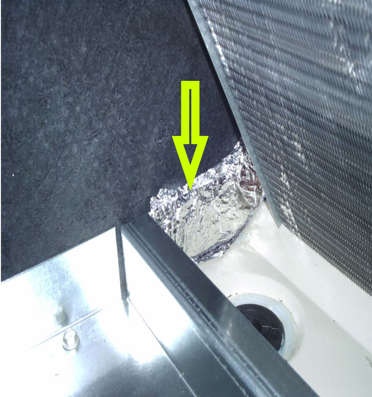
Cover caulking in drain pan with aluminum foil.
